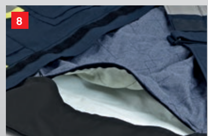
Inspection opening to check status of membranes
